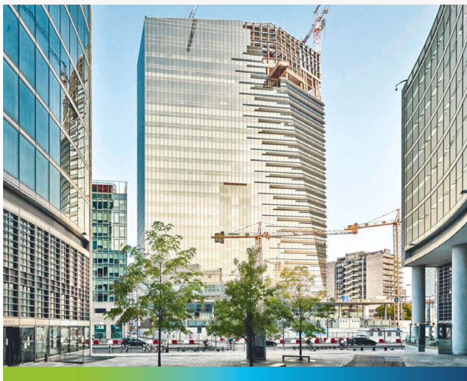
Gioia 22, in Milan's Porta Nuova former industrial district, is built with ECOPact green concrete with up to 50% lower CO 2
